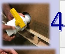
Thread the 2" ball valve assembly into the bottom 2" evacuation fitment. As the valve assembly is threaded into place, the increased thread engagement will cause the disposable cutter to pierce the membrane. Note: It is very important to thread the valve assembly all the way in to make sure the o-ring is seated and sealed against the evacuation fitment.
