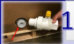
Remove the 2" screw cap from the bottom 2" flange on the bag liner.
