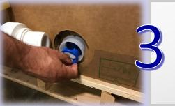
Take disposable ring cutter out of the evacuation fitment and turn the cutter around so the teeth are facing in (facing the membrane). Gently re-insert the cutter into the 2" evacuation.
