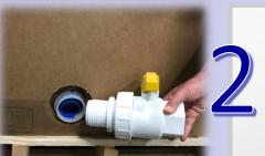
Make sure the valve is in the off position. The valve handle will be at a right angle (perpendicular) to the valve body.
