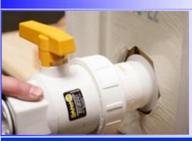
Close Valve and remove plunger cutter. You are now ready to connect to your hose for pumping
