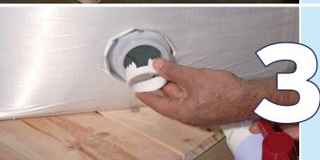
Take the disposable ring cutter and turn the cutter around so the teeth are facing the membrane. Gently reinsert the cutter into the 2" evacuation fitment.
